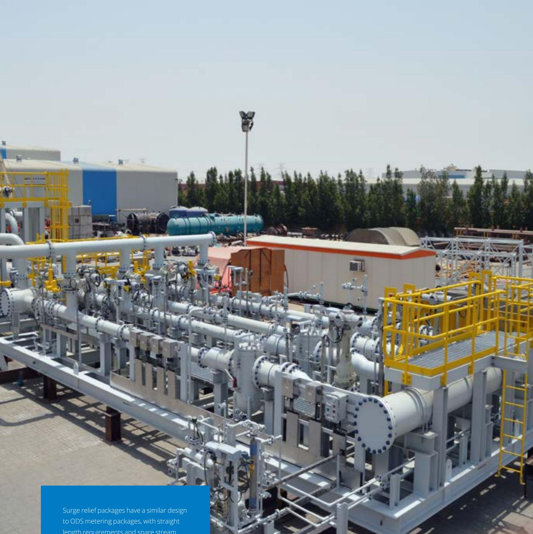
Surge relief packages have a similar design to ODS metering packages, with straight length requirements and spare stream capacity. Surge relief packages are rigid structure design with the isolation valves bolted directly to the structure.
